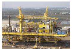
Project Description: The target of this project is to achieve the supply of 48 MW power in order to satisfy the electricity demand of the electric centrifugal pumps that PEMEX is installing to maximize the crude production in the Ku Maloob Zaap Field. The generation platform will be linked to the existing PB-ZAAP-C Production Complex using a bridge, and a submarine cable network; the peripheral platforms will be fed with 34.5 KW.
