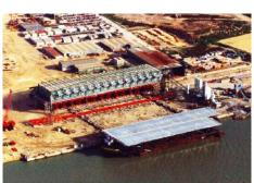
Scope of Work: Our SOW consisted on the construction engineering, procurement, fabrication, load out & transportation of the 49 spans of composite steel/concrete structure. The final dimensions of each span were 25 meters x 140 meters, with a final total weight for the 49 spans of 245,000 Tons. The transportation was performed in 25 shipments (every 21 days) with 2 spans per shipment with each span weighing approximately 5,000 tons.
