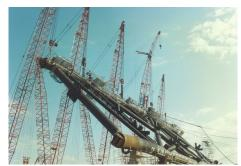
Scope of Work: Our SOW included the engineering, procurement, construction (EPC), load-out & sea fastening of the jacket with final dimensions of 146m  $\times$  40m  $\times$  40m and corresponding piles with a gross load out tonnage of 8,500 tons.
