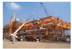
Project Description: The compression platform consists of an 8-leg jacket in 140 ft. water depth, supporting a 2-level process deck, compression modules containing Nuovo Pignone PGT25 turbine packages, Rolls Royce power generators and living quarters. The main compression platform is connected via a tripod-supported bridge to the existing AKAL GR Process Complex. It is also linked to a flare tripod via two bridges and an intermediate tripod.
